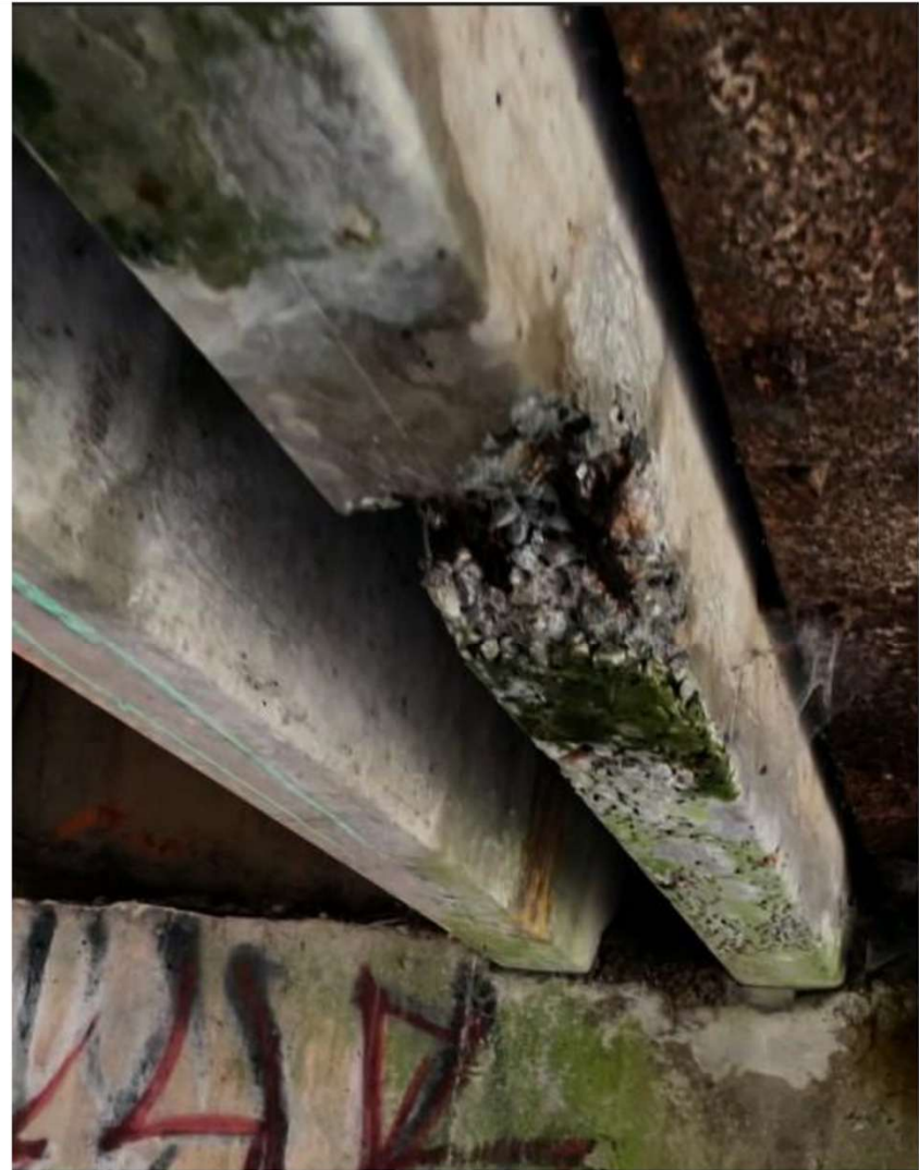
4 Girder A Spall in web 2 near Abutment 1. Both exposed strands are heavily corroded and ineffective.
